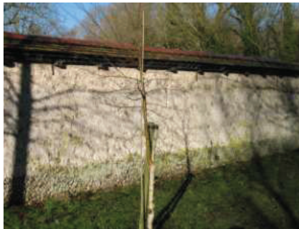
Photo 36: A retained cob wall in Byford Gardens, Porton
