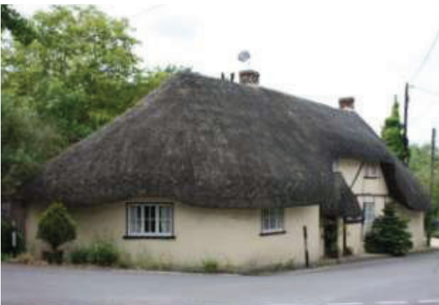
Photo 24: Thatch End, Church Road, Idmiston – colour-washed cob and brick under thatch
