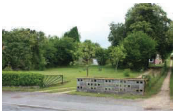
Photo 39: Inappropriate boundary treatment using concrete blocks in East Gomeldon
