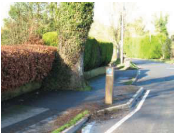
Photo 44: Winterslow Road pavement build out
