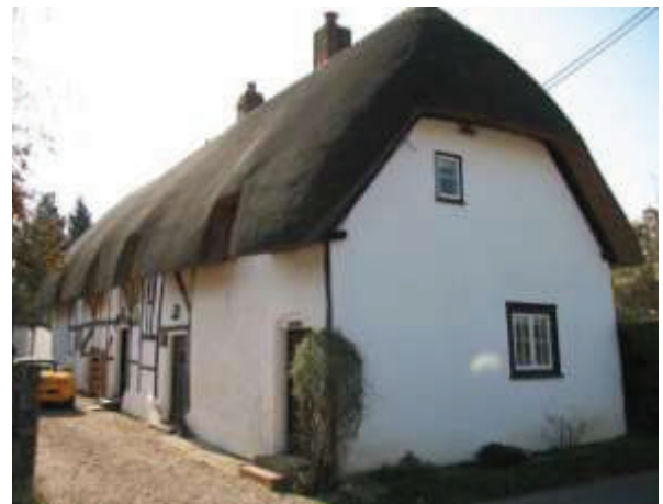
Photo 28: Ti Tree Cottage, High St, Porton - timber framed cottage extended in flint/cob under thatch
